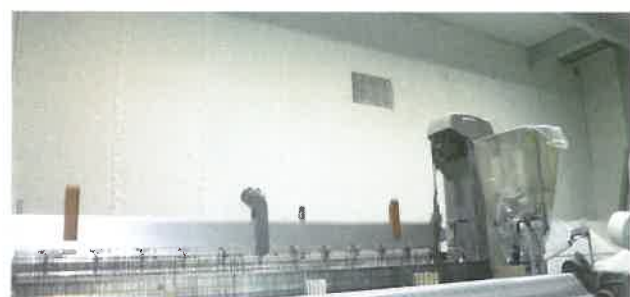
Real case using acoustic material (factory)
